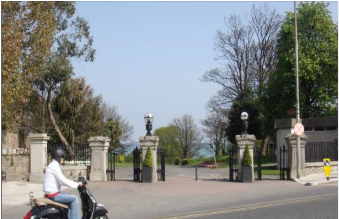
Plate 4.11 Entrance Gates, RPS 115
