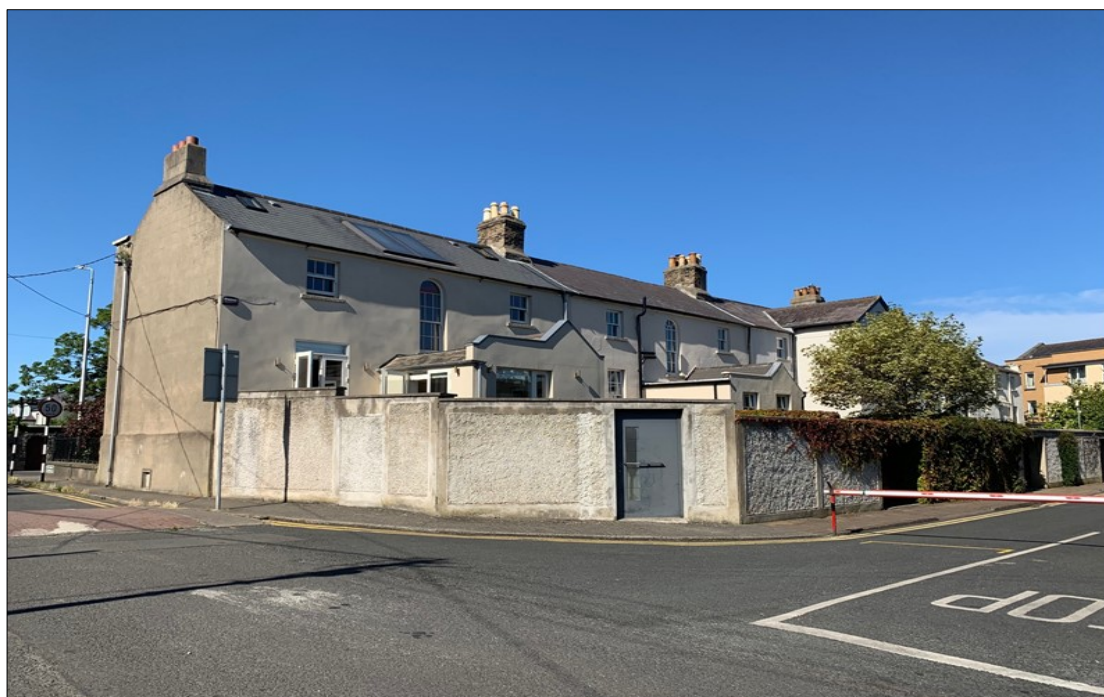
Plate 4.6 View of the rear of 8-16 Mt Merrion Avenue (even no's)
